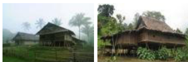
Figure 2. Traditional houses of Alifuru tribe from sago material in Selumena village (left) and in Binaiya mountain (right) (Source: Wijayanto, 2013)
