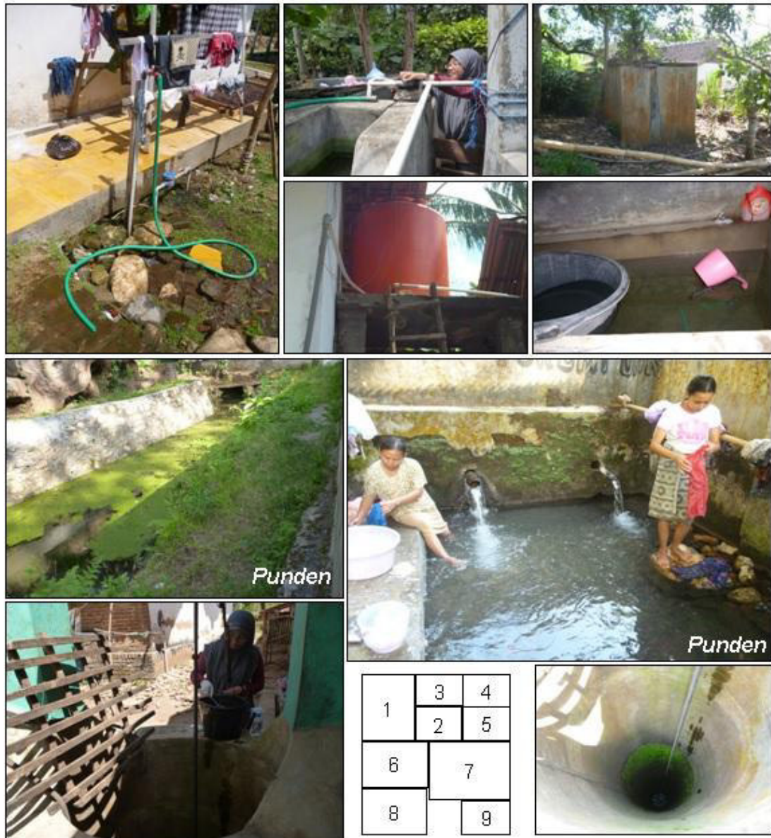
Fig. 2. Typical water facilities in the village. 1: Pipe water from faucet that water provided through local piping system without chlorination, 2: Water reservoir at a household, 3: Sampling of water from reservoir, 4: relay tank in the local pipe water system, 5: water in reservoir basin for washing use, 6: the source of river stream flow (punden: spring), 7: regiments' daily activity at spring (punden), 8: water sampling from a well, 9: inside of a well.
