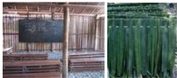
Figure 3. An example of how gaba-gaba can be used as interior in a school in South Seram (left) and the sago leaves as roof covering (Source: Almascatie, 2007)
